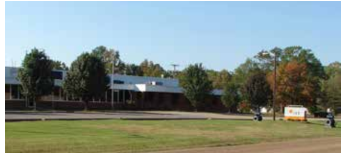
Amory, MS Facility
